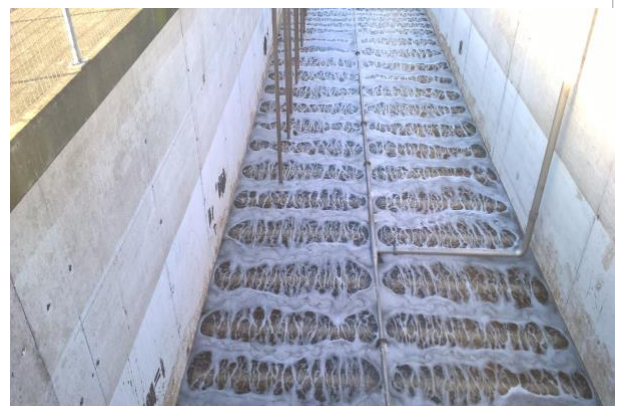
FBDA pattern test following installation
