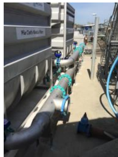
Joining pipe work for the site
