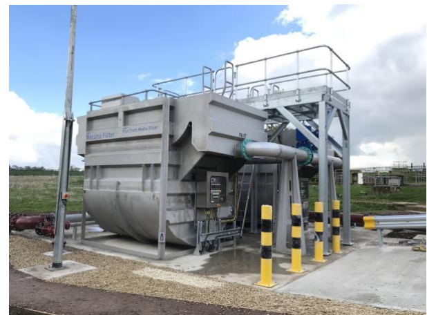
Woodstock STW • SF3/15-disc Filter Unit
